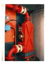
A picture of the electrolytic cell producing an antifouling solution to keep the sea chests and sea water circuits free from fouling.
